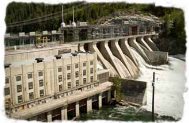
A hydro-electric dam in action
