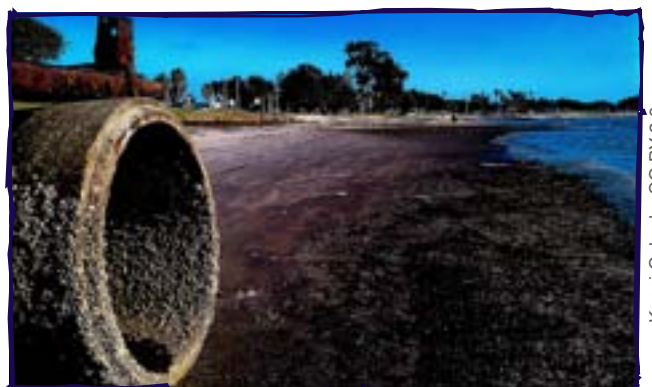
Combined sewage overflow pipe, San Diego
